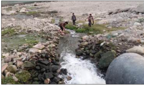
Image 7-4: Outlet of treated used water flowing into Ganga River
