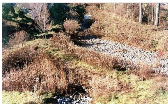
Image 7-24: Infiltration trenches
