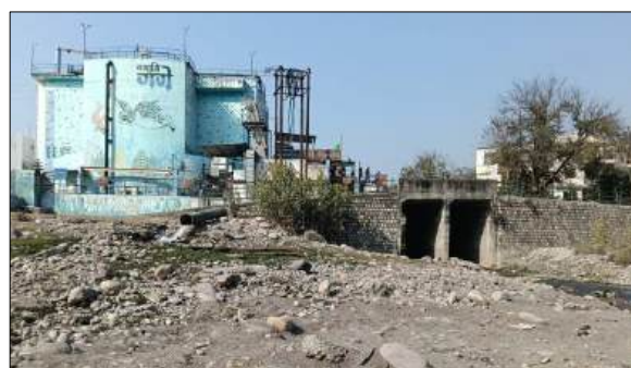
Image 7-2: Chandreshwar Nagar 7.5 MLD STP and dhalwala nallah outflow point
